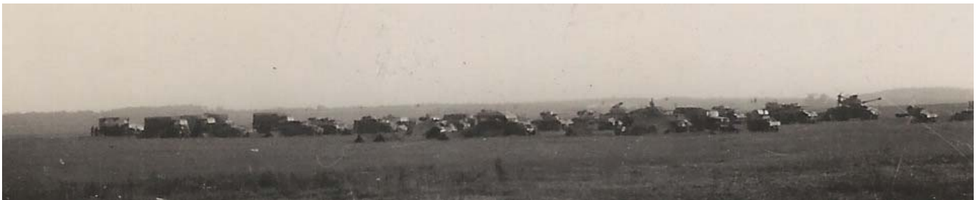
Photo Courtesy of Photographer 2nd Lieutenant Stuart Ruthven Description: The Sabre Squadron at Marienthal Austria, overnight harbour Date: Circa 1945-1946
